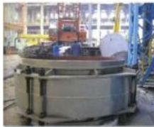
The installation site of the compensator with the main hot tube of 1260m 3 blast furnace
