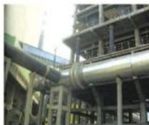
The installation site of compensator with gas tube of blast furnace
