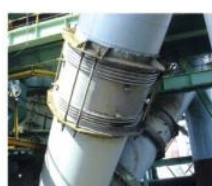
The using site of gas riser compensator
